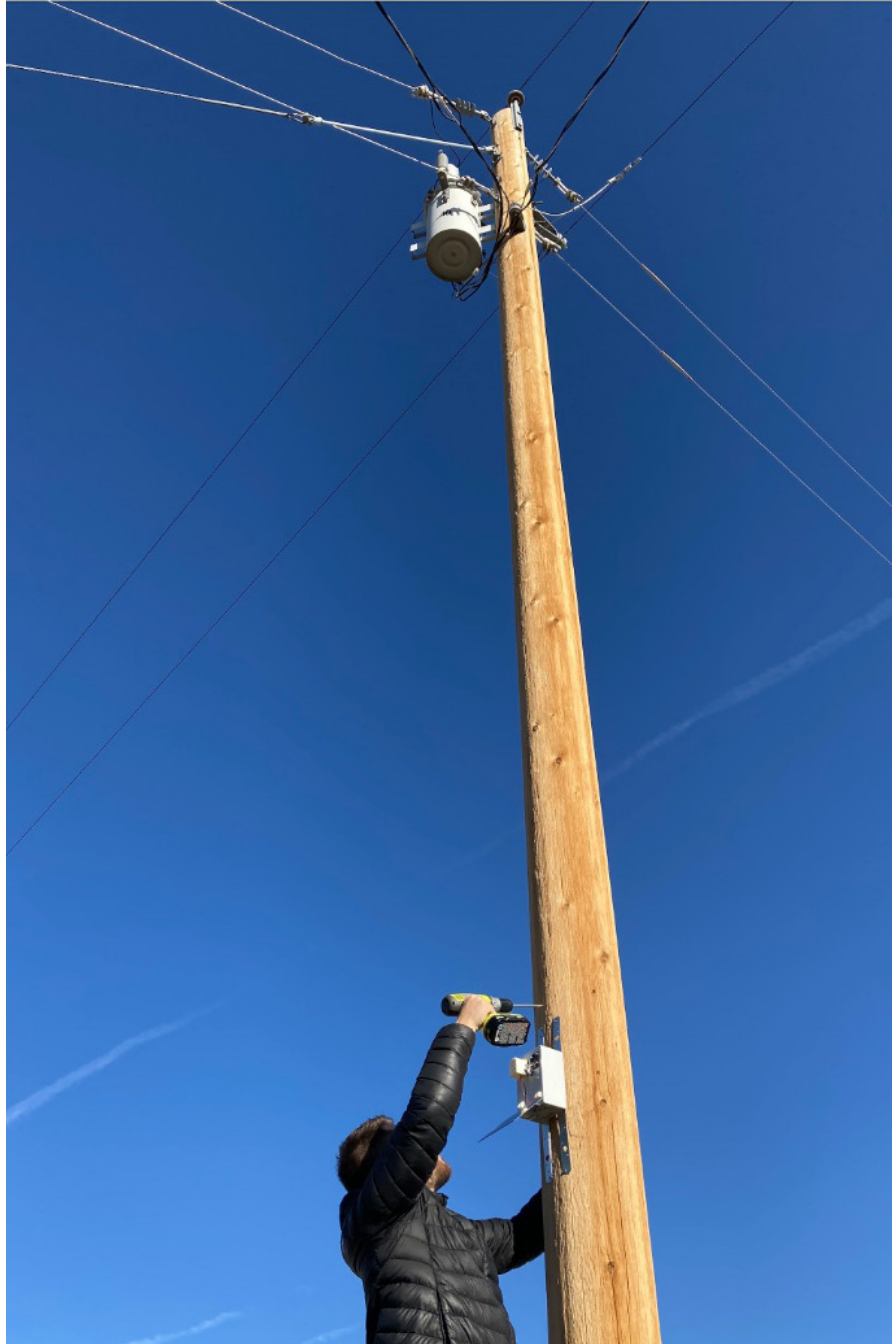
Gridware's Co-Founder and CEO, Timothy Barat, installing their first unit on a service utility pole. Gridware is developing industrial internet of things (IOT) systems and risk simulation software for utilities that own and maintain electricity distribution grids that will monitor poles, conductors, and equipment to predict where they may fail and ignite a wildfire.
